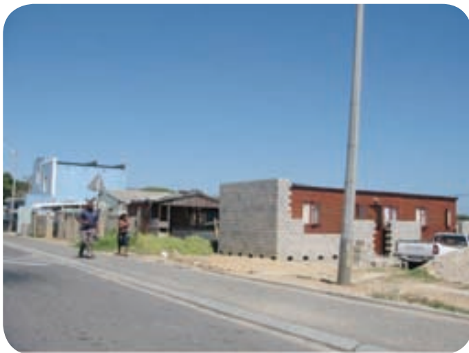
Many builders site their 'Wendyhouse' (temporary wooden lodging- a house within a home) on foundations and over time as savings are made build a house around it.
