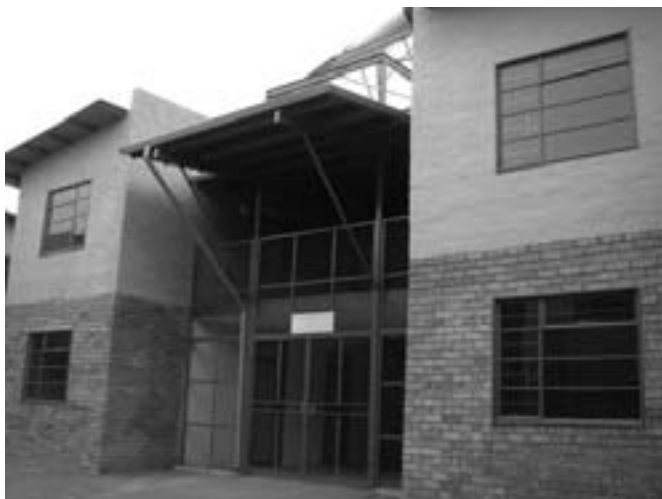
Photo 10. Housing Managed by JOSHCO in Alexandra
